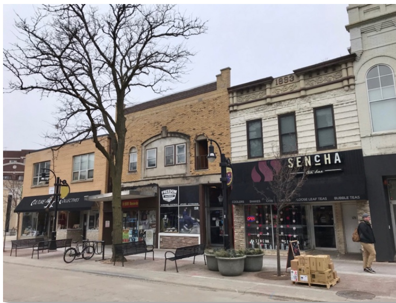
Three buildings on the 400 block of State Street
