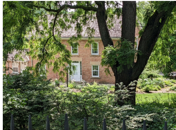
View of front of OST and landmarked west yard from Council Crest. The proposed house would block this view.
